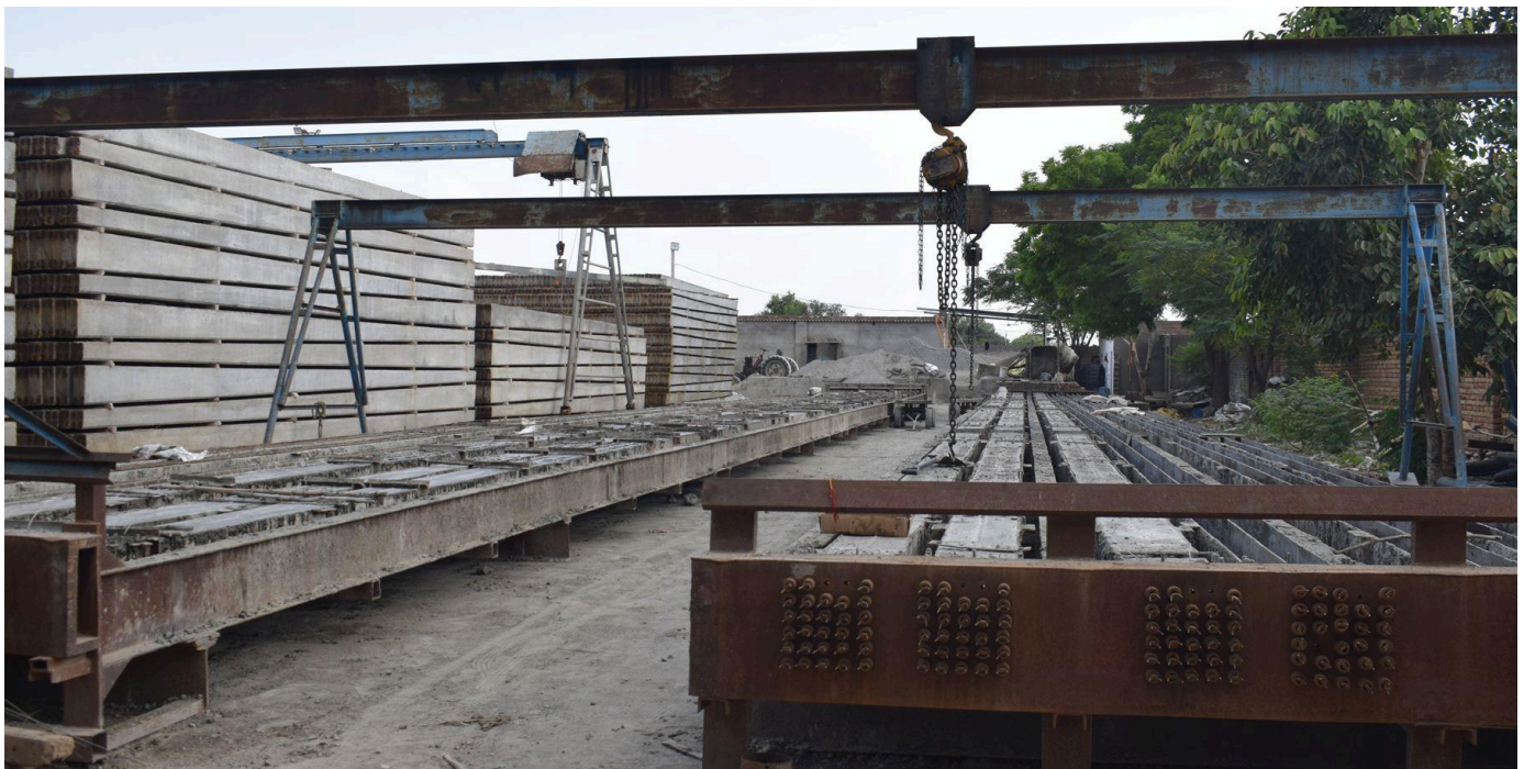
Pole casting beds under the gantry
