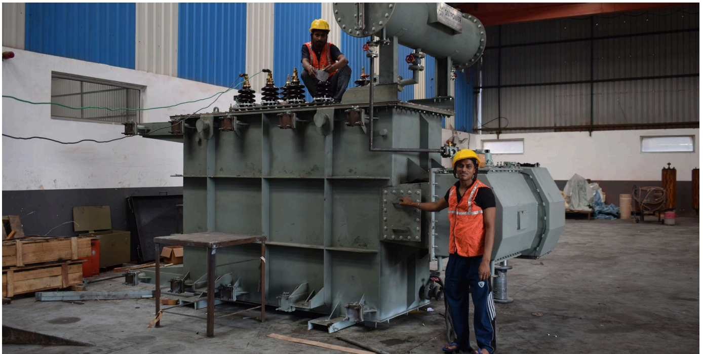
Power transformer under assembly
